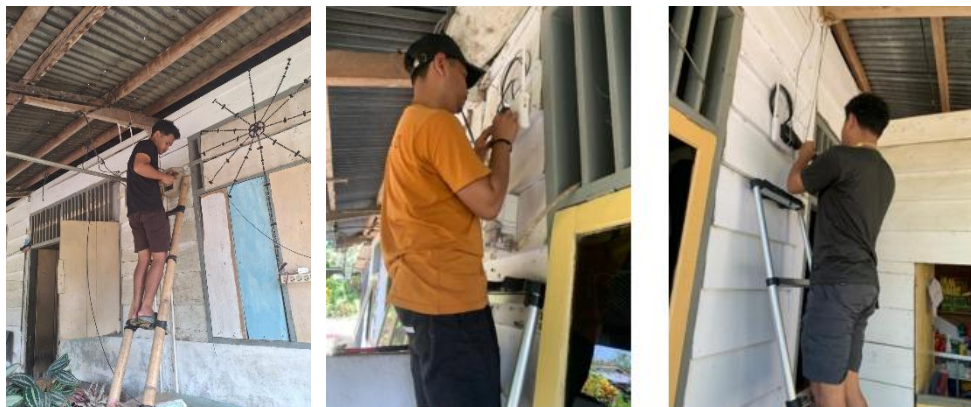
Figure 9. Access Point Installation.
